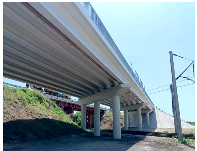
Restoration of a bridge in the Kharkiv region
